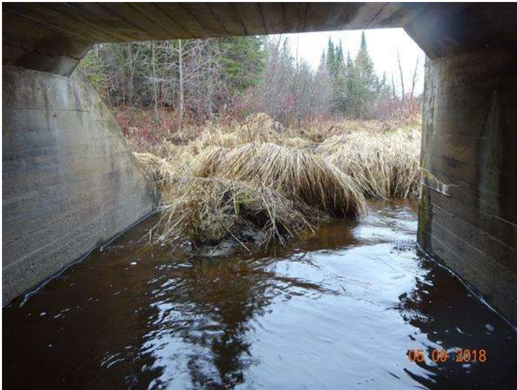
Photo 27 - Barrel 1 Inlet Blockage
