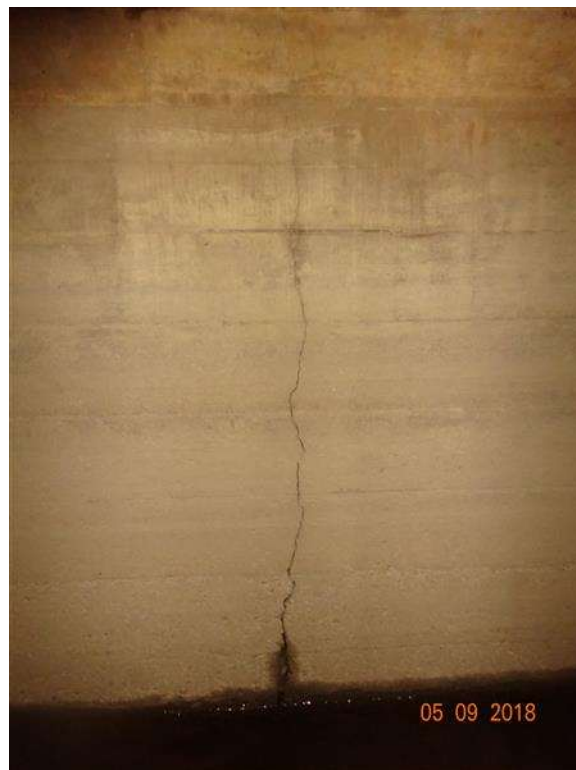
Photo 12 - Barrel Vertical Crack
