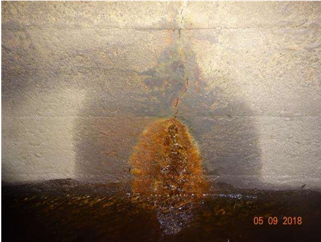
Photo 11 - Barrel 2 East Wall Crack Leaching With Rust Staining
