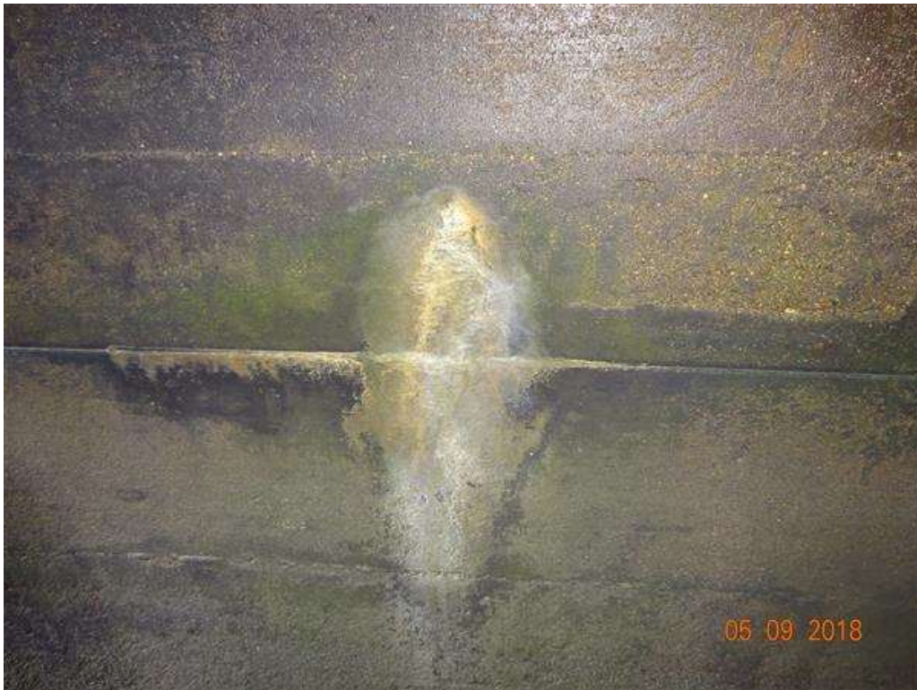
Photo 16 - Barrel Wall Form Tie Hole Leaching
