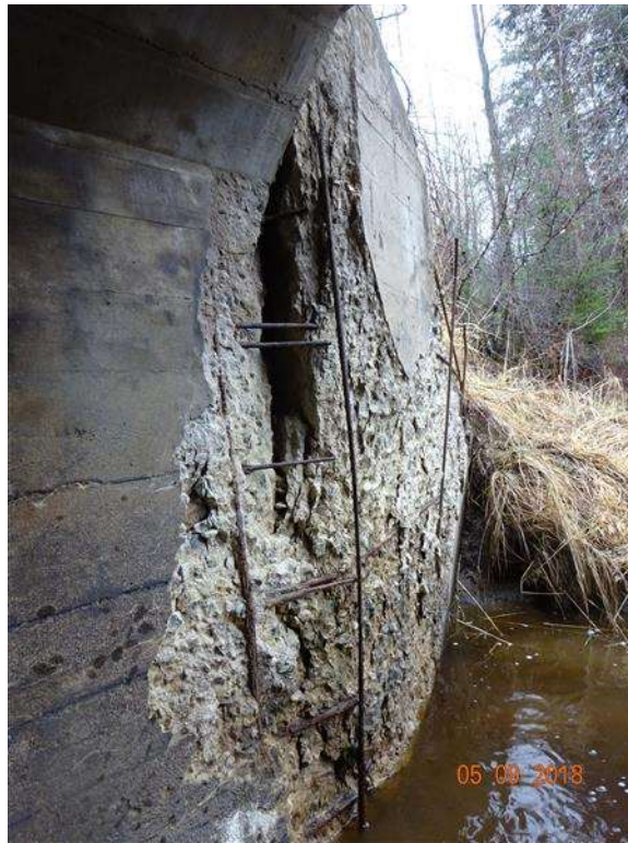
Photo 20 - SE Wing and Barrel Connection Failure
