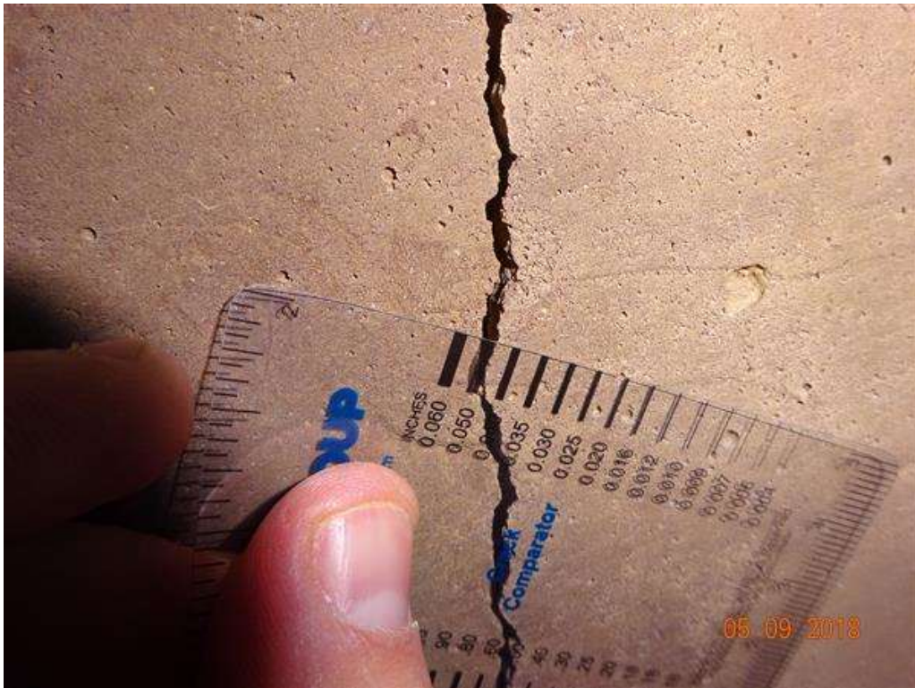
Photo 14 - Barrel Vertical Crack 0.05in
