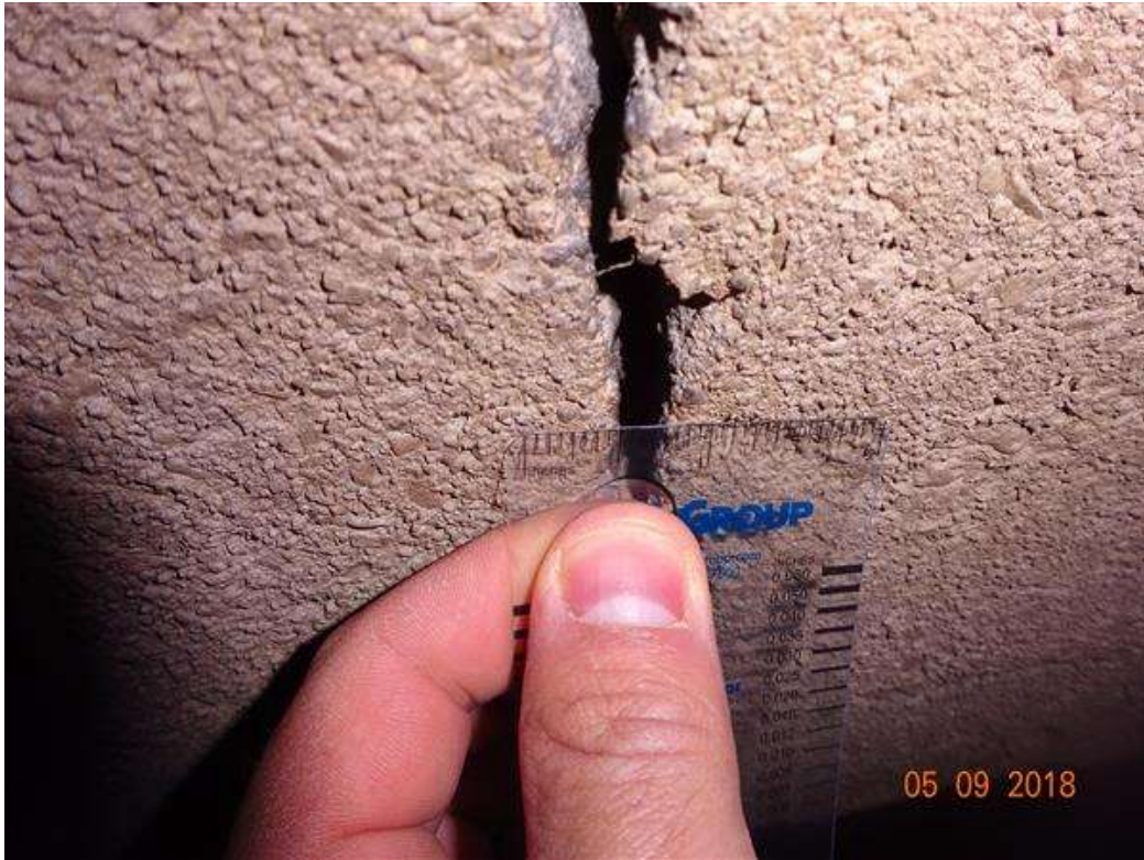
Photo 15 - Barrel Vertical Crack 0.25in at Bottom of Wall
