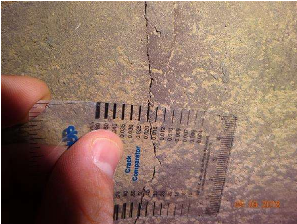
Photo 13 - Barrel Vertical Crack Width 0.02in
